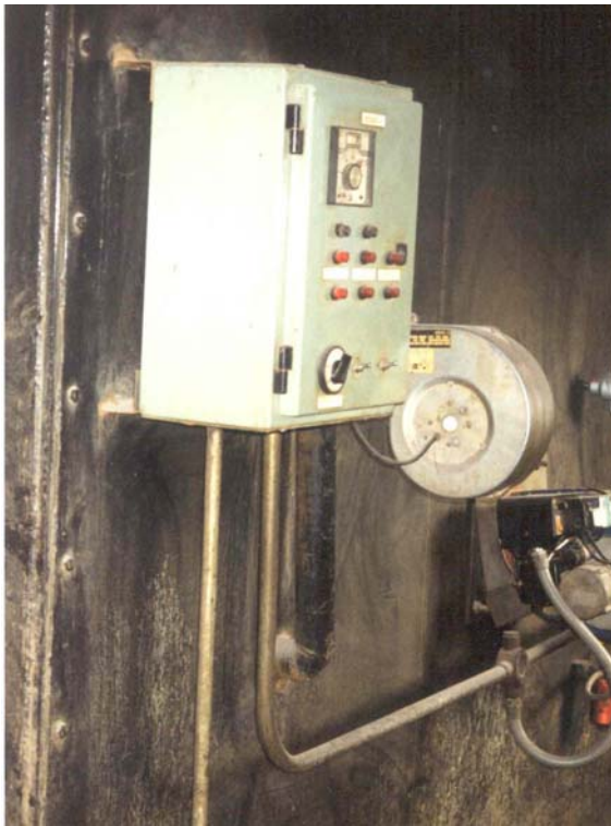
Abb. 21 Instrument panel of a health-care waste incinerator
