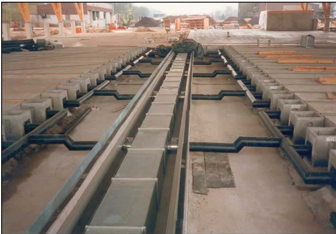
Fig. 5.28: Configuration of a Sealed Decomposition Area (Heidenheimer decomposition plates) (Photo: Ingenieurgesellschaft Abfall)
